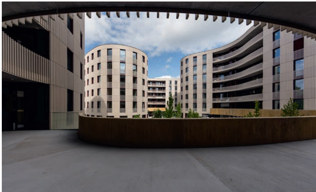
The student residence Swiss Life completed in 2016 is Minergie-P-Eco certified and uses ground-source heat pumps. © ETH Zürich/Alessandro Della Bella
